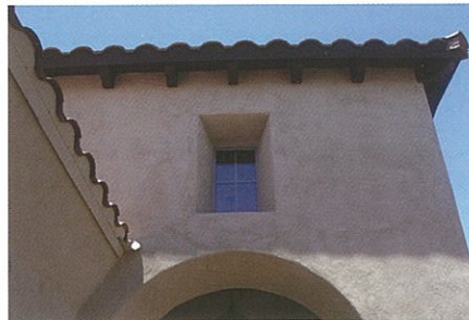
Simple, sculpted forms define a Spanish Colonial elevation. Note the use of exposed rafter tails, in tandem with coved stucco fascia.
